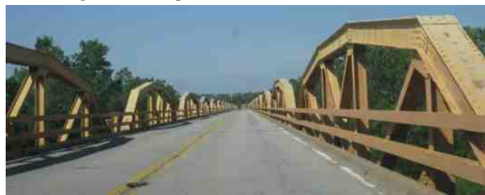
"Pony Bridge" over "South Canadian River".
