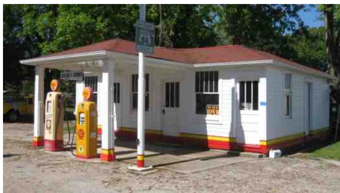
Flot restaureret "Shell" tankstation i Mount Olive.
